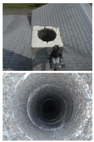
**CONDITION:** Deteriorated mortar, Advise spot tuck pointing also Unlined flue, Recommend repair and further inspection prior to use. Patch cracks in chimney cap.
