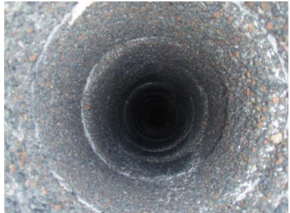
**CONDITION:** Deteriorated mortar, Advise spot tuck pointing also Unlined flue, Recommend repair and further inspection prior to use. Patch cracks in chimney cap.
