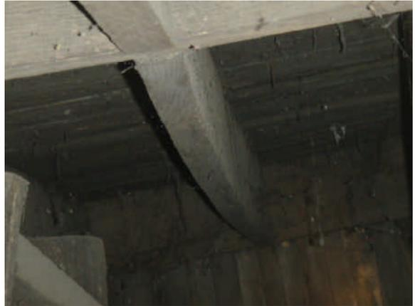
**FLOOR JOISTS:** Floor joists are sagging/cracked. Moisture/Rot noted.
